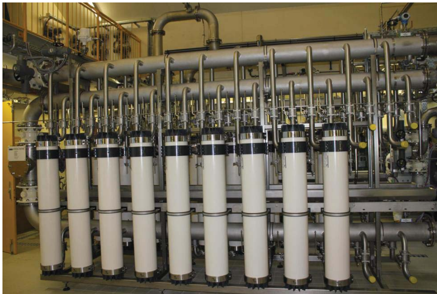
Bildunterschrift: Clean drinking water for the city of Luxembourg thanks to cutting-edge ultrafiltration technology
